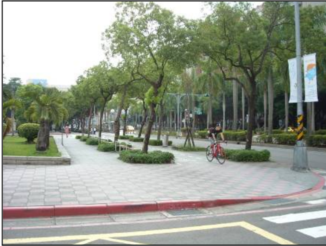
Setup wheelchair ramps
