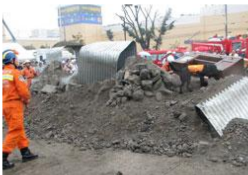
Rescue dogs from Taipei at work at collapse site
